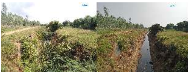
Noyyal Cannel After Cleaning Debris and Bushes
