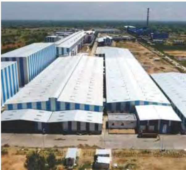
TNPL's Board Plant - Unit II
