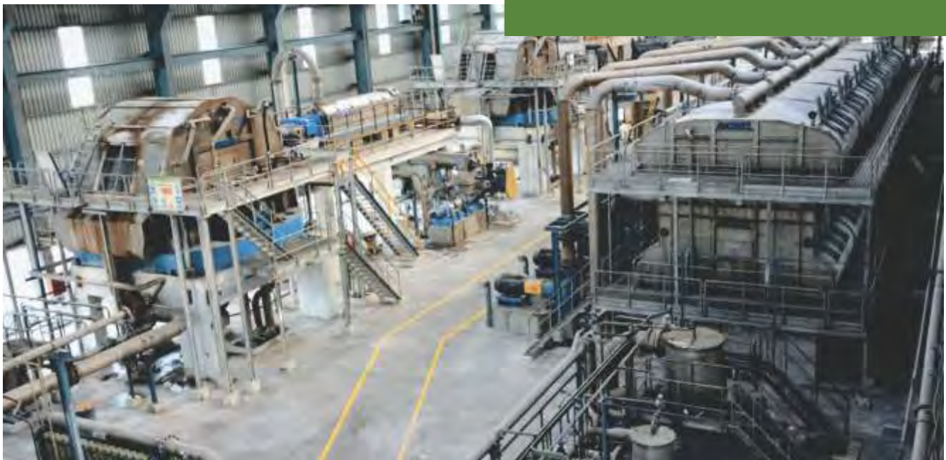
State of the art Deinked Pulp line in TNPL Paper Mill - Unit I
