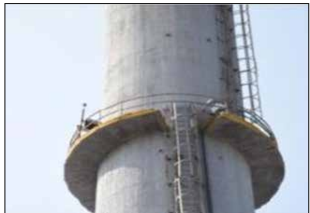
Continuous Stack Emission Monitoring Station
