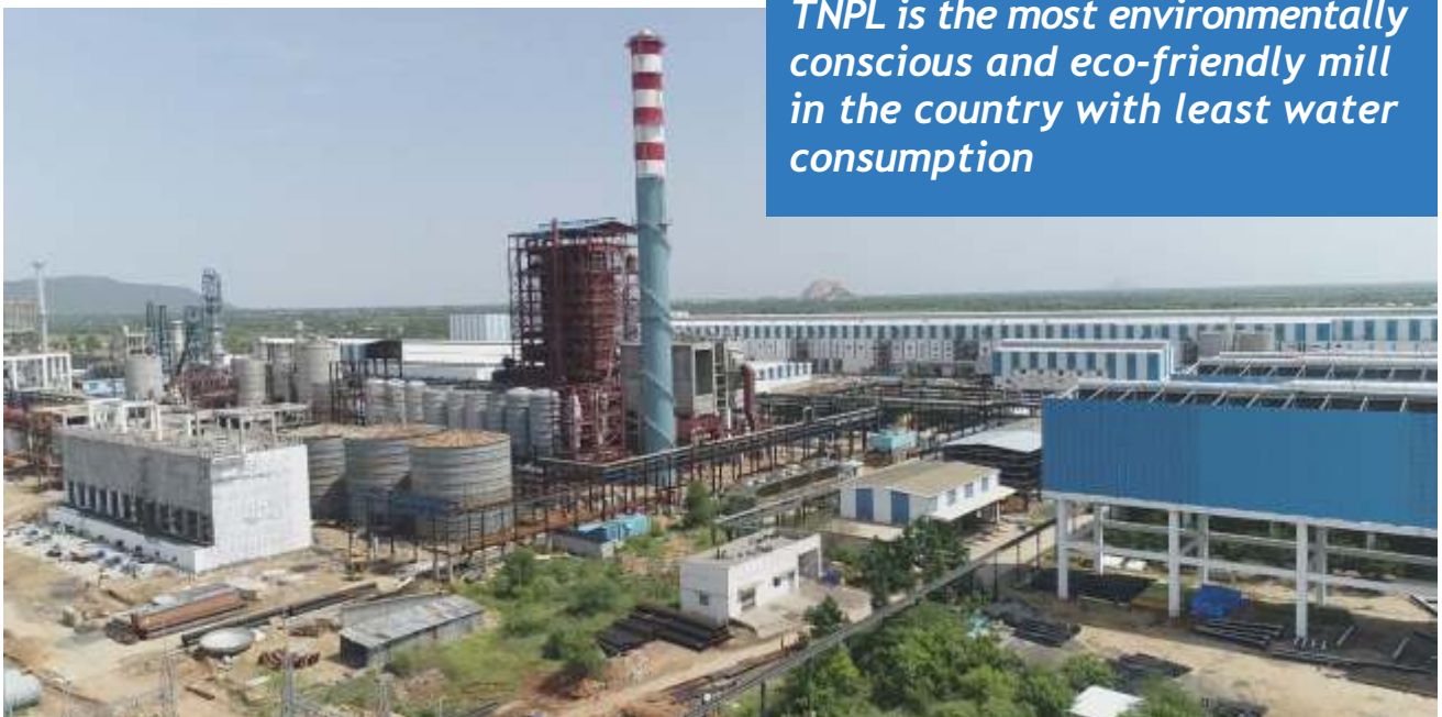
Mill Expansion Plan of Unit II - Erection of Chemical Recovery Boiler in progress
