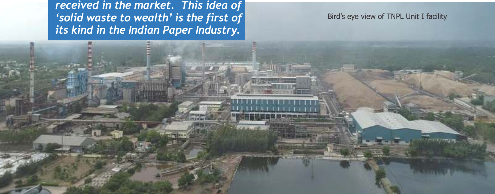
Project Site - Mill Expansion Plan in Unit II under implementation
