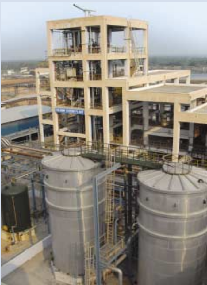
The new 15 tpd Chlorine di-oxide plant
