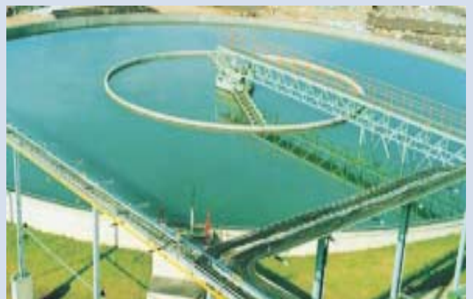
Effluent Treatment Plant
