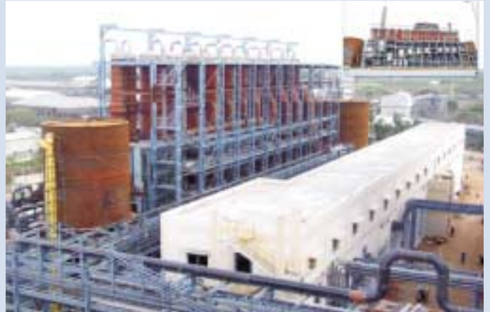
The new Ten body, Seven Effect Free Flow Falling Film Evaporation Plant, the largest black liquor evaporation plant in India
