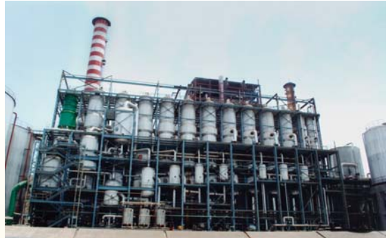
Multiple effect evaporator
