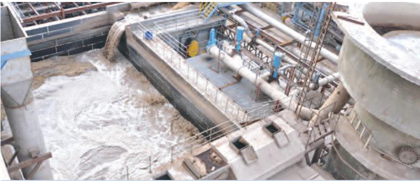
CBP III - Reclaim and Bagasse Washing
