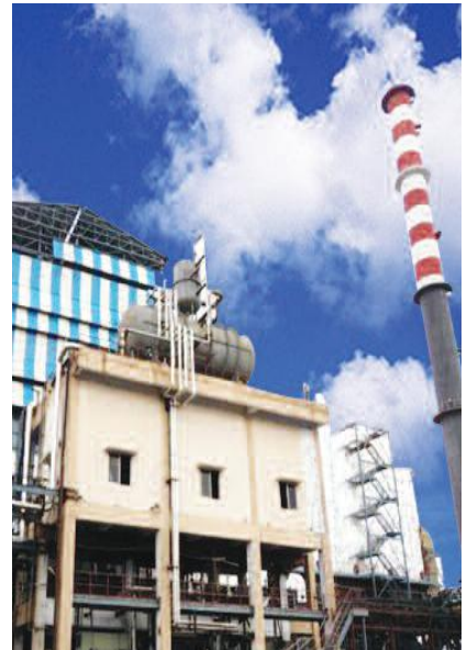
125 TPH Power Boiler No.6
