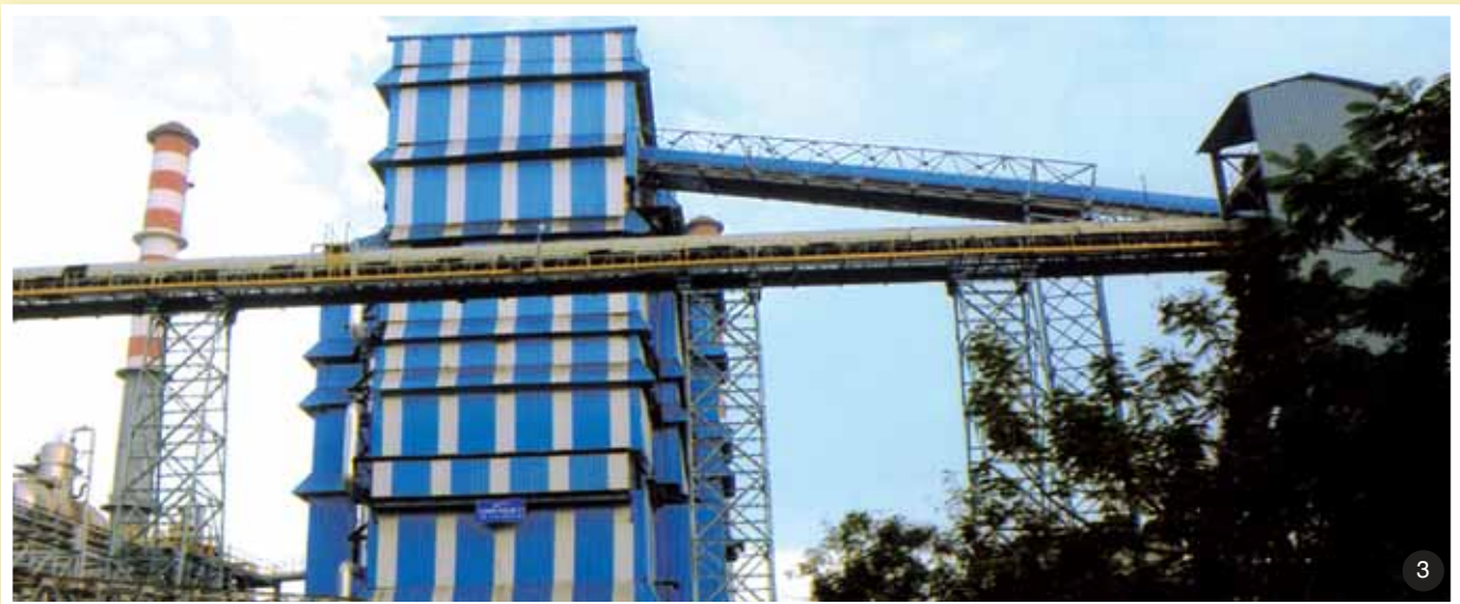
(1) Cement Plant (2) DIP - De-inking Plant (3) 125 Tonnes per hour Boiler
