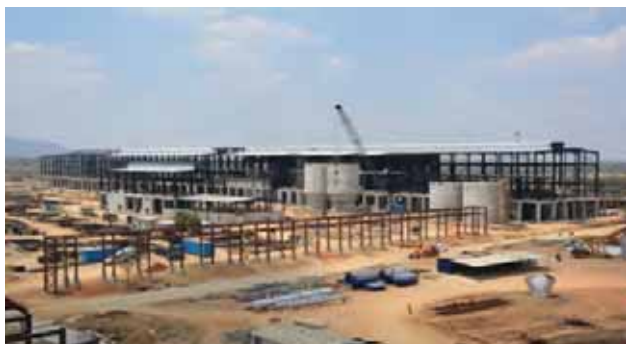
Board Machine Construction – Bird's eye view
