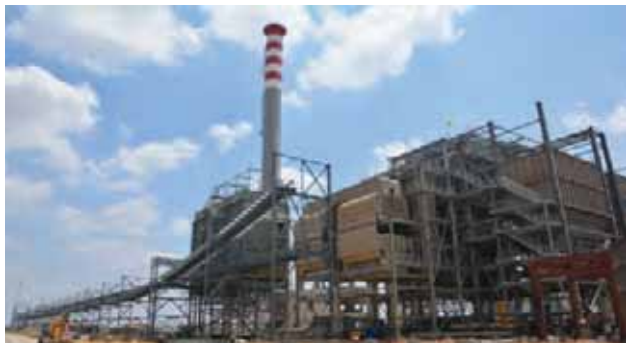
Boiler erection in progress
