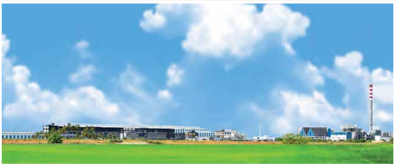
Panoramic view of the Board Plant under Construction
